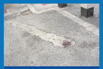
STORM WATER INTAKE APPEARS INADEQUATE
