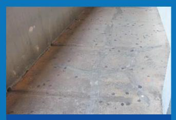
FLOOR SLAB – REPAIRED CRACKS
