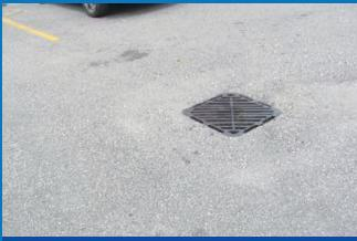
STORM WATER INTAKE APPEARS INADEQUATE
