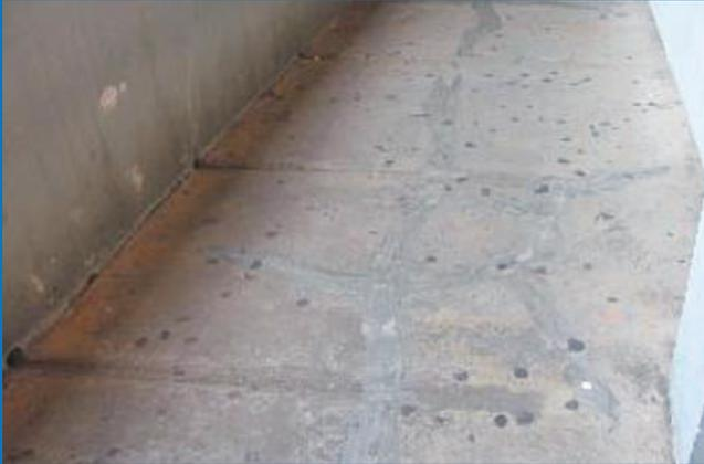
■ FLOOR SLAB – REPAIRED CRACKS
