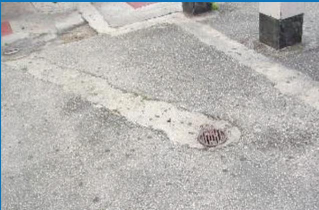
■ STORM WATER INTAKE APPEARS INADEQUATE
