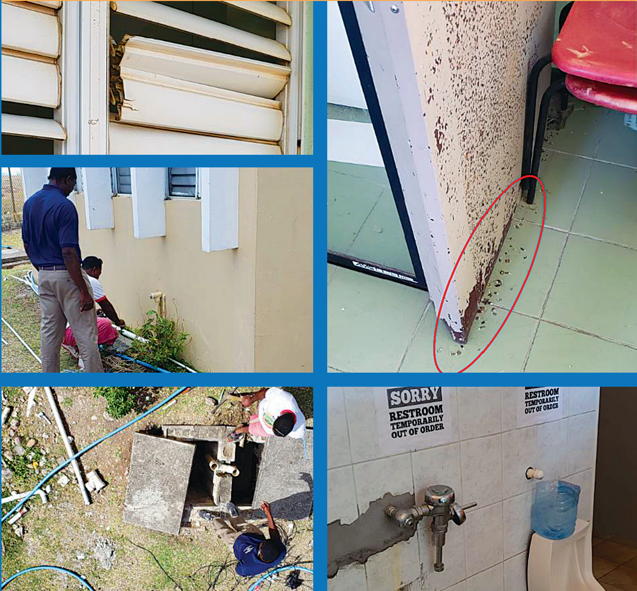
FIGURE 7.2: AREAS FOR IMPROVEMENT IDENTIFIED
