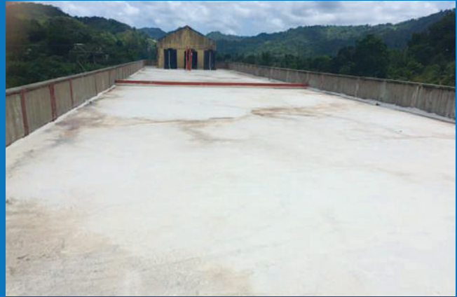
■ ROOF RECENTLY REPAIRED
