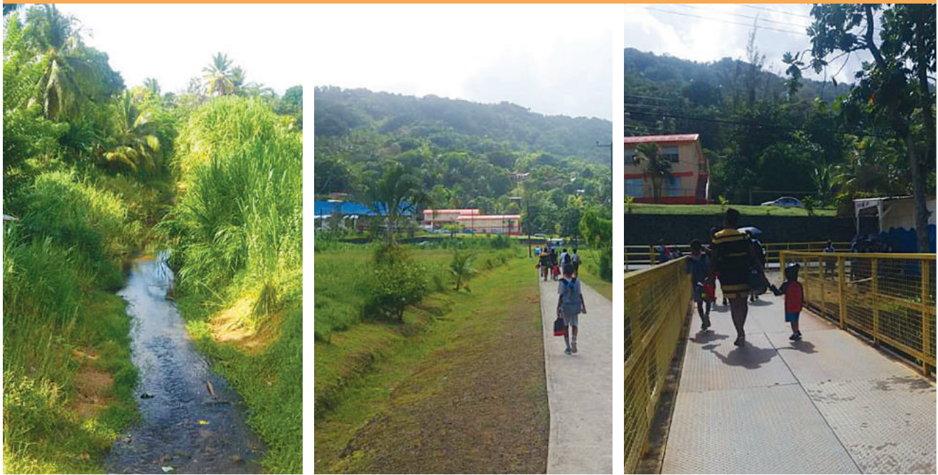
FIGURE 4.2: IMAGES OF BEXON PRIMARY – STUDENTS AND STAFF MUST CROSS FLOOD PRONE AREAS TO ACCESS MAIN ROAD
