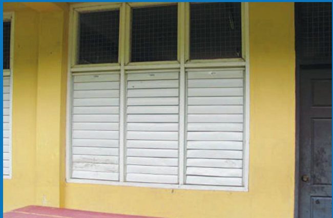
■ TYPICAL ALUMINIUM LOUVRE
