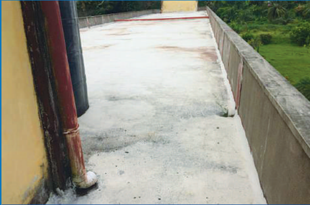
■ ROOF RECENTLY REPAIRED
