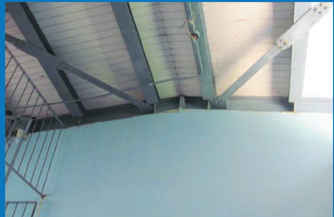
■ STRUCTURAL STEEL FRAME BUILDING IN REASONABLY GOOD CONDITION
