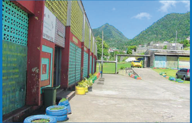
■ FRONT FAÇADE OF BUILDING
