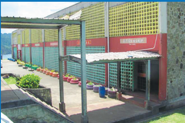
■ FRONT FAÇADE OF BUILDING
