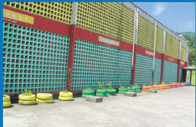
■ FRONT FAÇADE OF BUILDING
