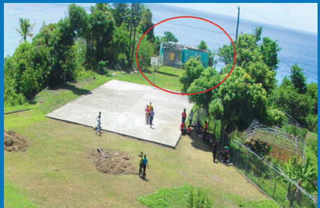
■ BUILDING WHOSE EXTERNAL WALL FAILED UNDER HURRICANE FORCE WINDS
