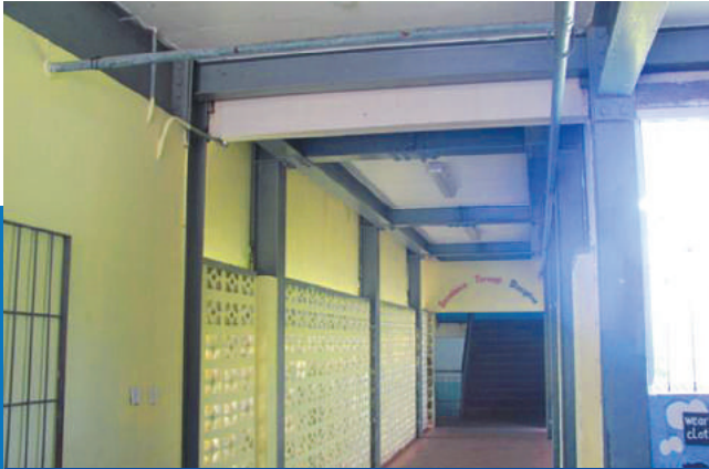
■ STRUCTURAL STEEL FRAME BUILDING IN REASONABLY GOOD CONDITION
