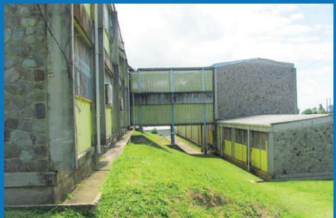
■ VIEW OF MULTI-LEVEL, COVERED, ENCLOSED LINK-BRIDGE BETWEEN CLASSROOM BLOCKS
