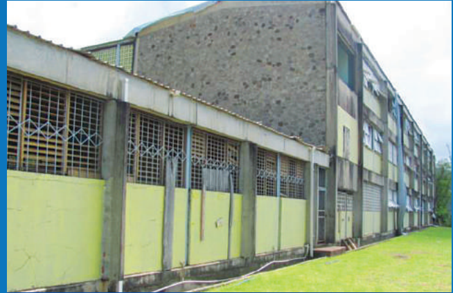
■ REAR ELEVATION OF BUILDING
