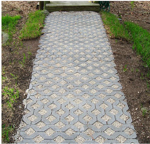
Figure 5: Installed Permeable Pavers
