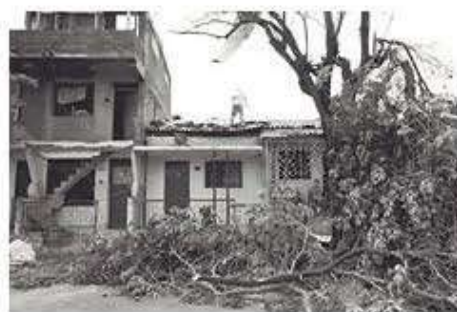
Figure 3.2: Collapse caused by Hurricane Sandy's winds.
