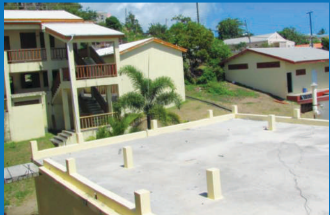
■ BUILDING WITH CONCRETE ROOF
