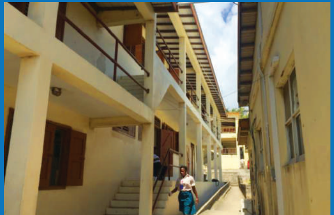
■ NARROW PASSAGES - CONSEQUENCE OF UNPLANNED INCREMENTAL CONSTRUCTION
