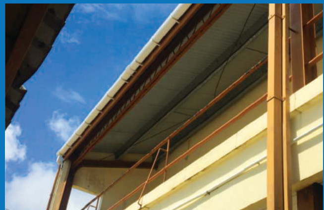
■ STRUCTURAL STEEL FRAME BUILDING
