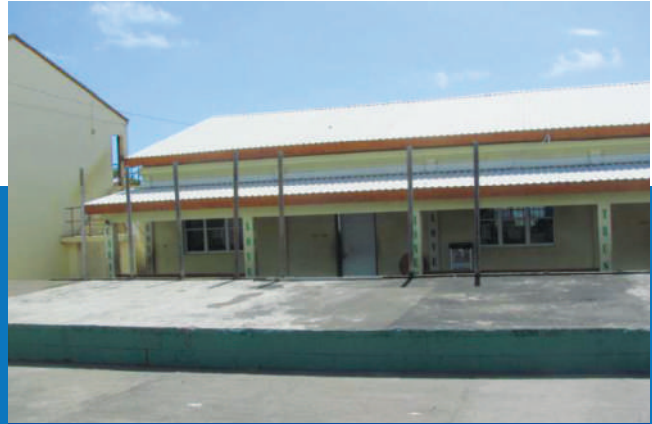
■ SINGLE STOREY ADMINISTRATIVE BUILDING
