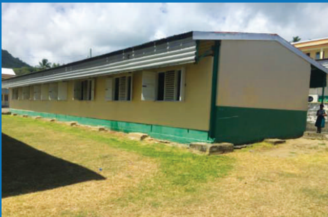
■ SINGLE STOREY CLASSROOM BLOCK
