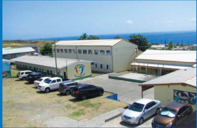
■ PANORAMIC VIEW - SECTIONS OF COMPOUND
