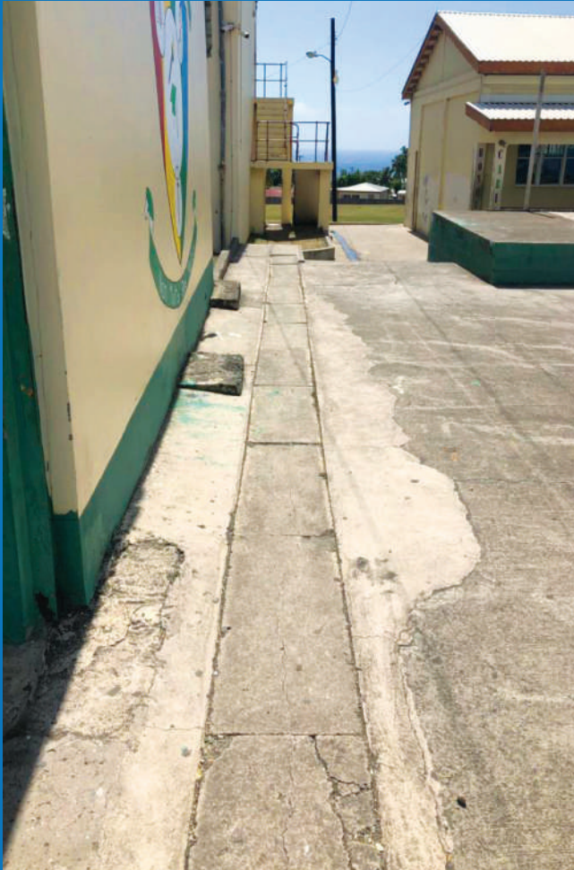
■ DRAINS - PART OF EXTERNAL DRAINAGE NETWORK
