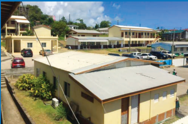
■ PANORAMIC VIEW - SECTIONS OF COMPOUND
