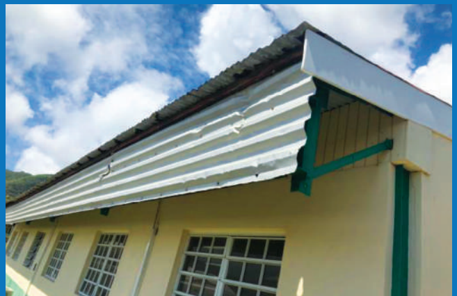
■ MAKESHIFT SUN AND RAIN BARRIER – VERTICAL ALUZINC SHEETS
