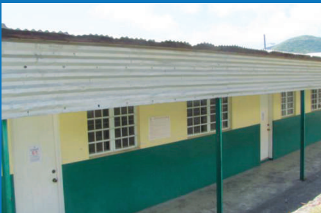
■ MAKESHIFT SUN AND RAIN BARRIER – VERTICAL ALUZINC SHEETS
