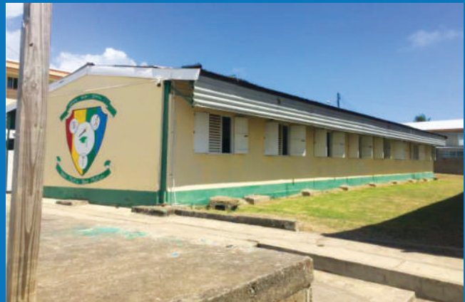
■ SINGLE STOREY CLASSROOM BLOCK
