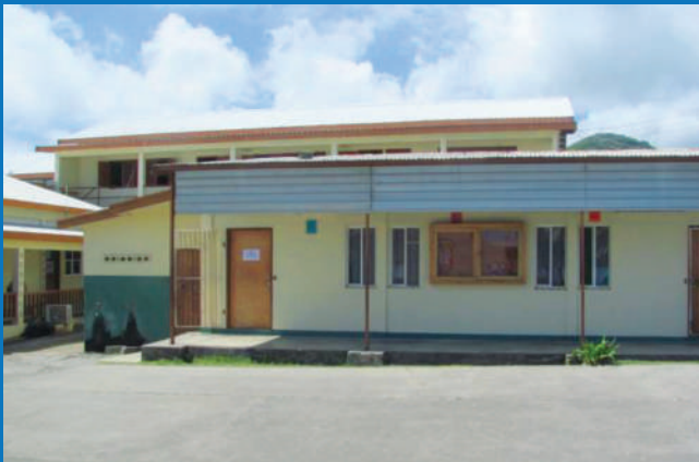
■ SINGLE STOREY ADMINISTRATIVE BUILDING
