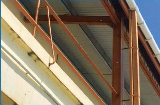
■ STRUCTURAL STEEL FRAME BUILDING
