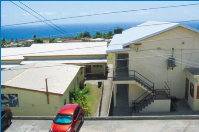
■ PANORAMIC VIEW - SECTIONS OF COMPOUND
