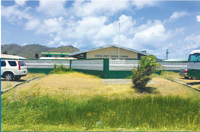
■ PARTIAL VIEW OF COMPOUND
