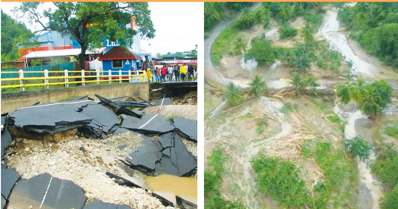
FIGURE 3.1: IMPACTS OF HURRICANE TOMAS (2010). SOURCE: SLU DRR
