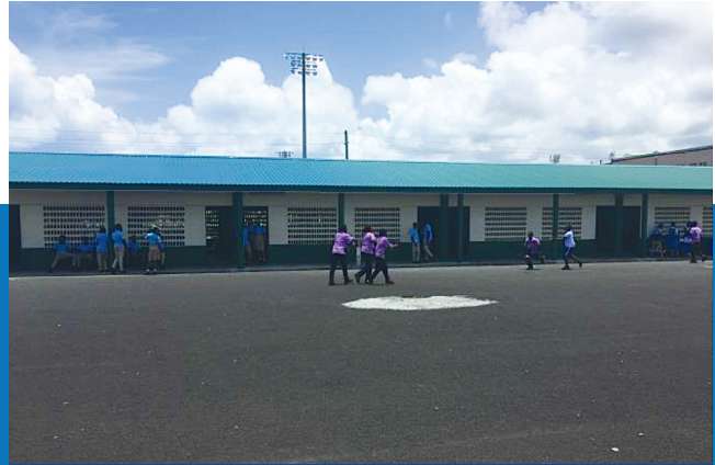
■ BUILDING WITH VENT BLOCKS - NEW ROOF
