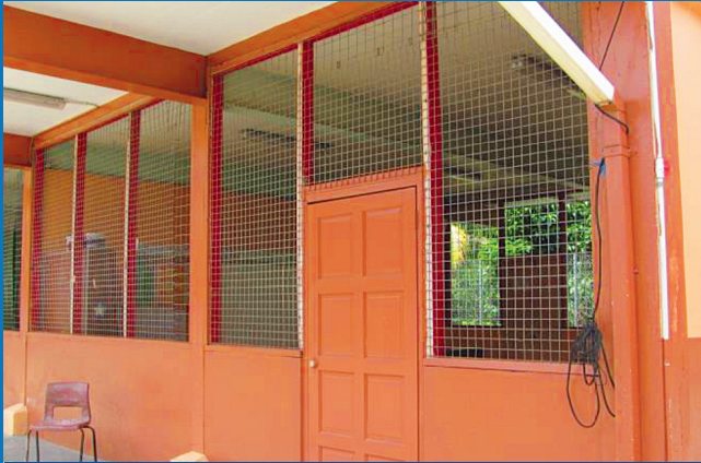
■ STRUCTURAL STEEL FRAME, WIRE-MESH WALLS, WOODEN
