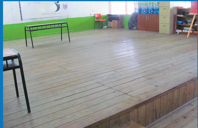
■ UPPER LEVEL TIMBER FLOOR
