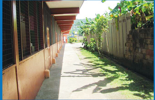
■ STRUCTURAL STEEL FRAME, WIRE-MESH WALLS, WOODEN
