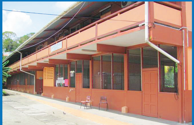
■ STRUCTURAL STEEL FRAME, WIRE-MESH WALLS, WOODEN
