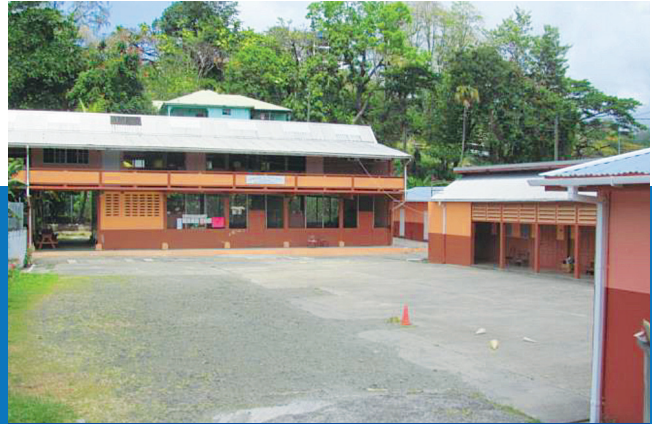
■ MAIN COMPOUND SHOWING GATHERING/ ASSEMBLY AREA
