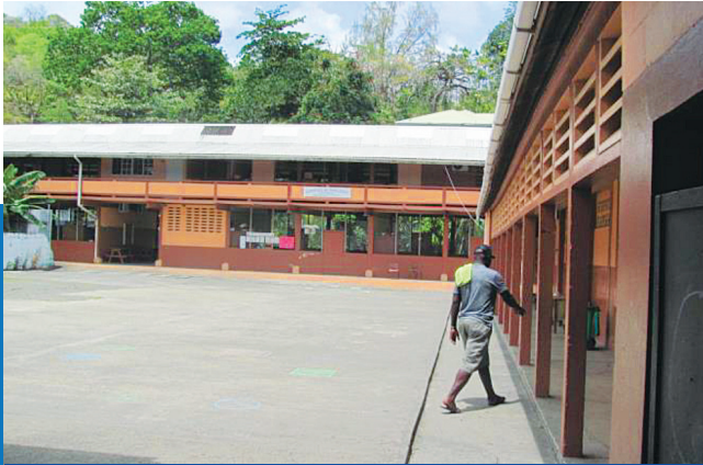
■ MAIN COMPOUND SHOWING GATHERING/ ASSEMBLY AREA
