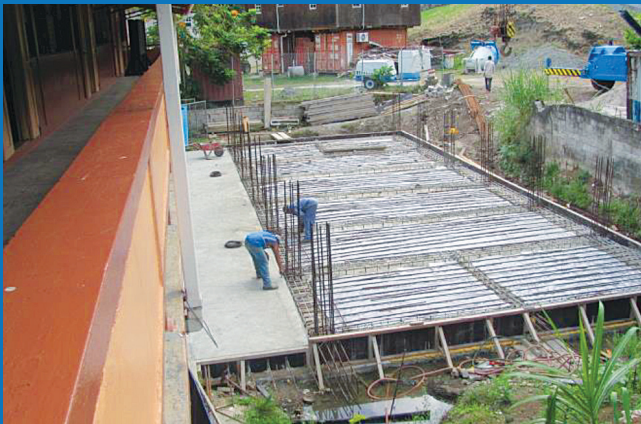
■ EXPANSION IN PROGRESS
