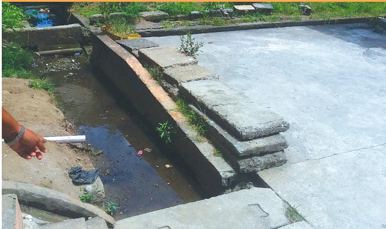
FIGURE 4.1: PORTION OF COMMUNITY DRAIN RUNNING THROUGH THE SCHOOL (SOURCE: CHARIM.NET)
