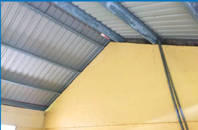
■ ROOF OVER STAIRWELL
