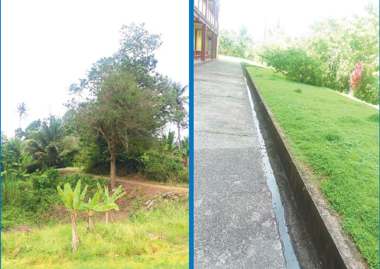
FIGURE 7.1: SELECTED PICTURES OF BEXON PRIMARY SHOWING SOME KEY AREAS FOR IMPROVEMENT (LEFT TO RIGHT: STEEP ACCESS ROAD USED AS EVACUATION ROUTE, SHALLOW DRAINS FOR HANDLING STORM WATER)
