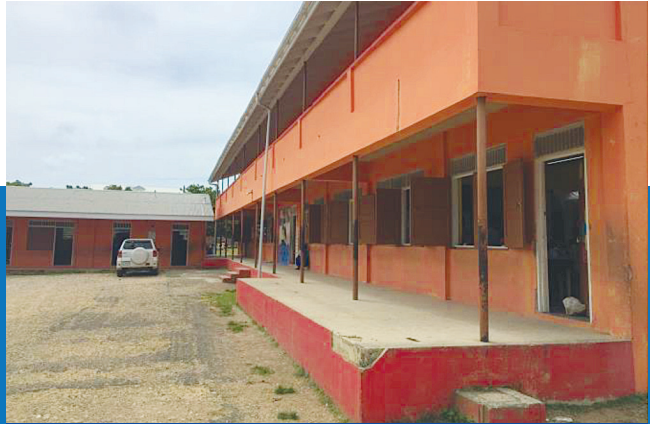
■ MAIN CLASSROOM BLOCK #1 - FRONT ELEVATION
