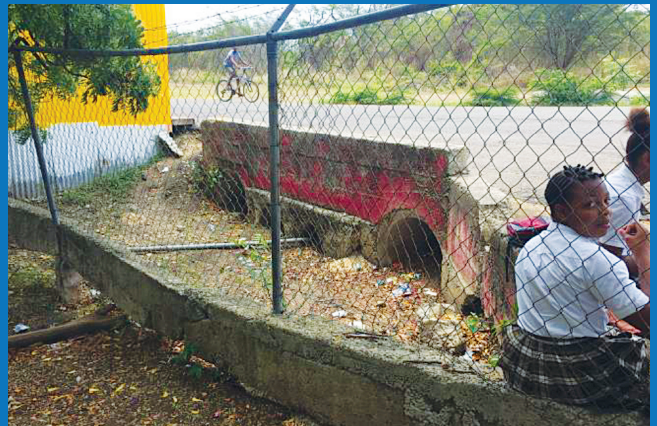
■ MAJOR WATERWAY FLOWS THROUGH SCHOOL COMPOUND IN SHALLOW DITCH
