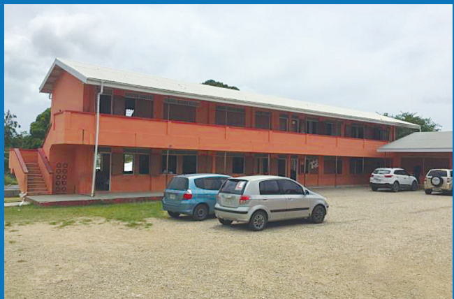
■ MAIN CLASSROOM BLOCK #2 - FRONT ELEVATION
