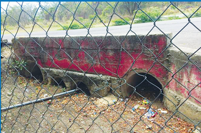
■ MAJOR WATERWAY FLOWS THROUGH SCHOOL COMPOUND IN SHALLOW DITCH
