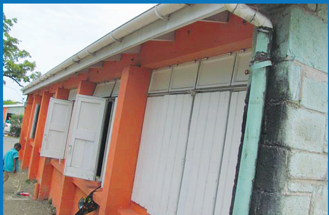
■ ONE OF THE ORIGINAL BUILDINGS IN NEED OF REFURBISHMENT
