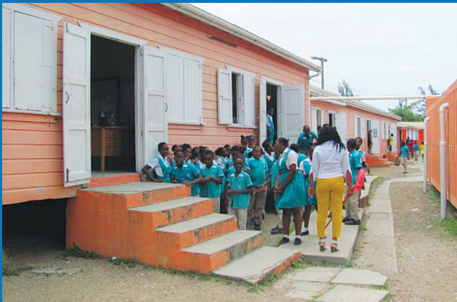
■ TIMBER BUILDING REMAINS VERY VULNERABLE TO HURRICANES
