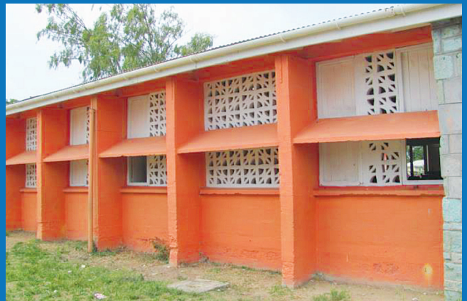
■ STYLIZED BREEZE BLOCKS AND WOODEN WINDOWS
