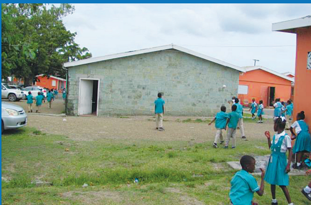
■ ONE OF THE ORIGINAL BUILDINGS IN NEED OF REFURBISHMENT
