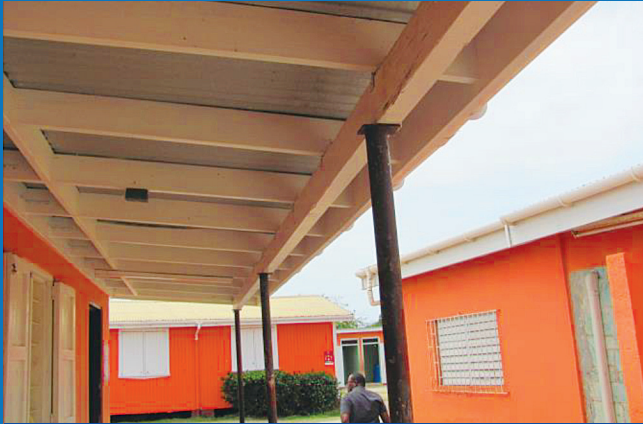
■ KITCHEN ROOF STRUCTURE ANCHORED WITH METAL STRAPS
