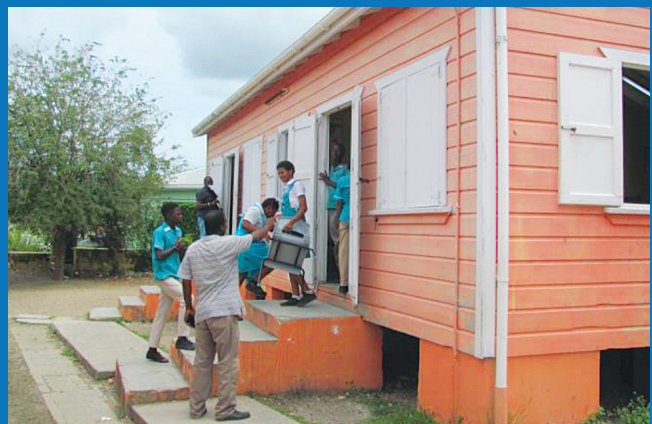
■ TIMBER BUILDING REMAINS VERY VULNERABLE TO HURRICANES
