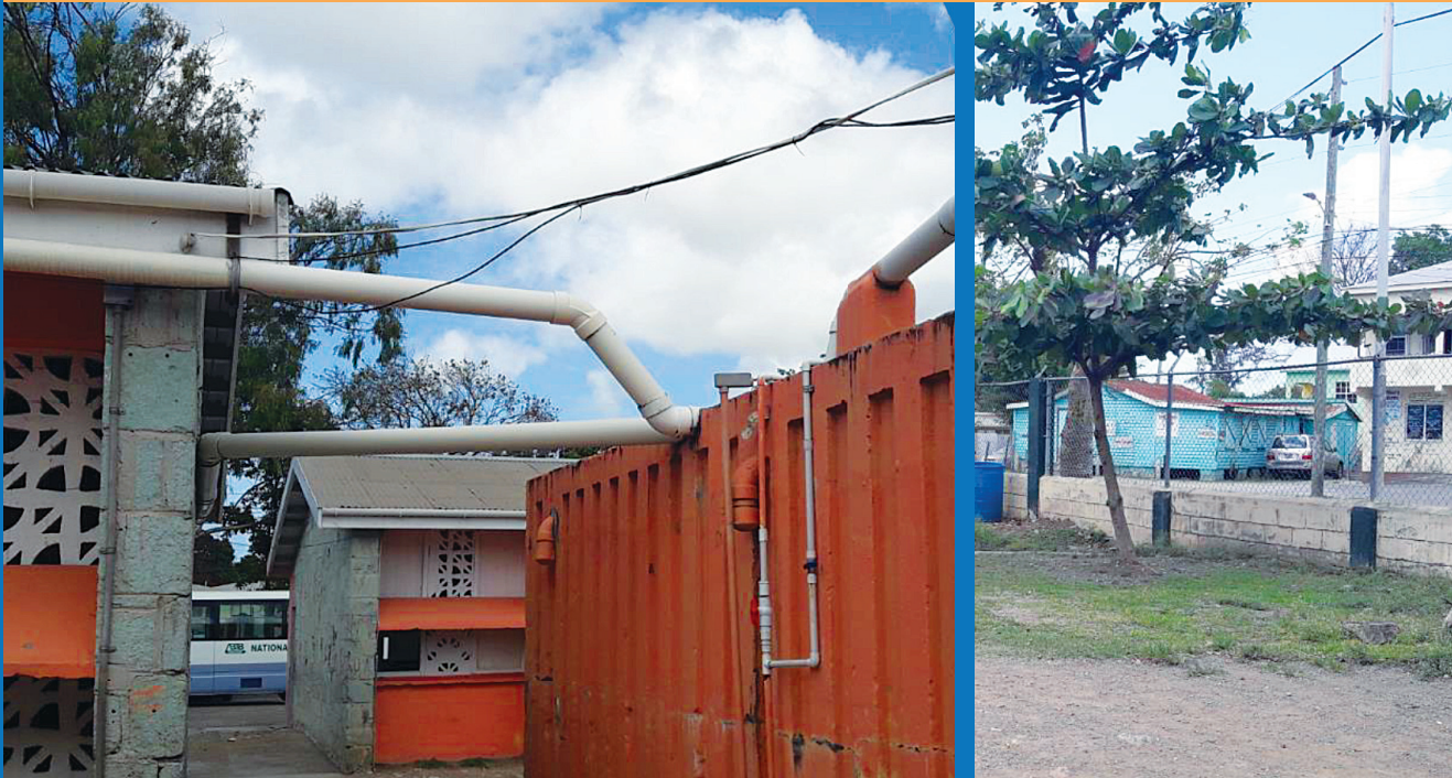
FIGURE 7.1: SOME EXAMPLES OF KEY STRENGTHS AT THE GOLDEN GROVE PRIMARY SCHOOL (RAINWATER HARVESTING AND RECYCLING)
