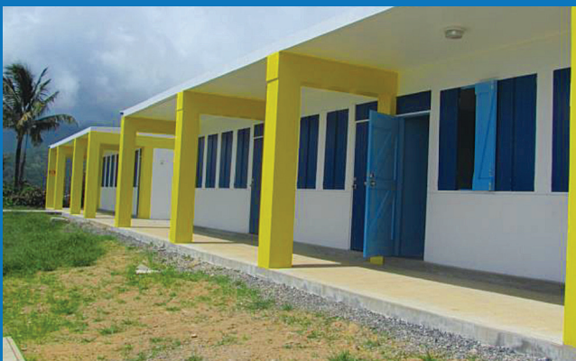
NEW BLOCK UNDER CONSTRUCTION
