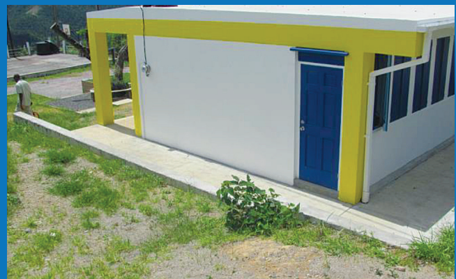
NEW BLOCK UNDER CONSTRUCTION
