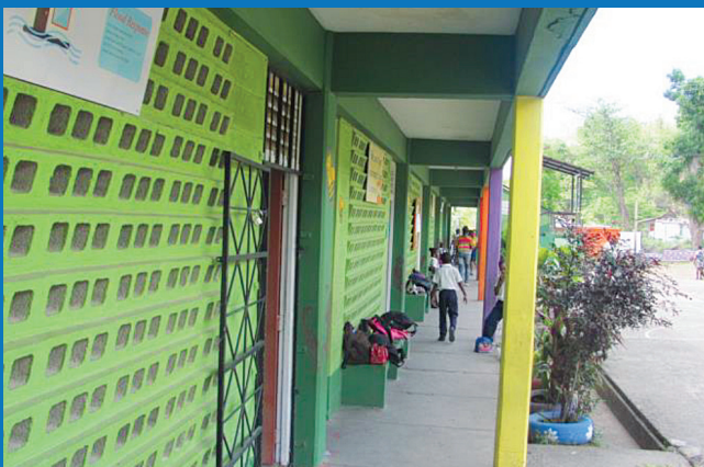
GROUND FLOOR WALKWAY
