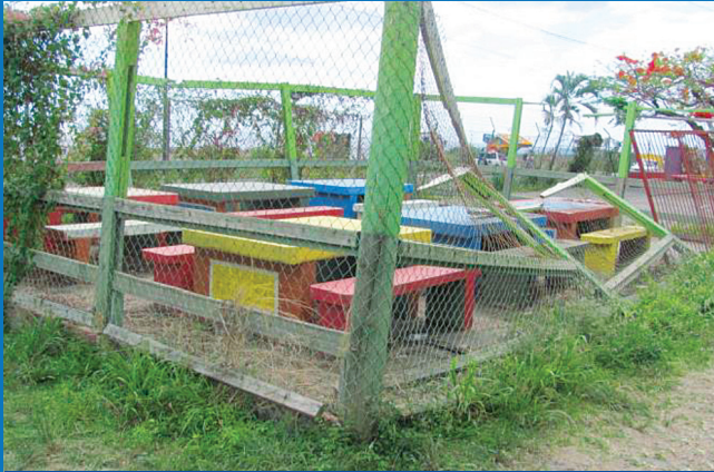
■ LUNCH ROOM BEFORE HURRICANE
