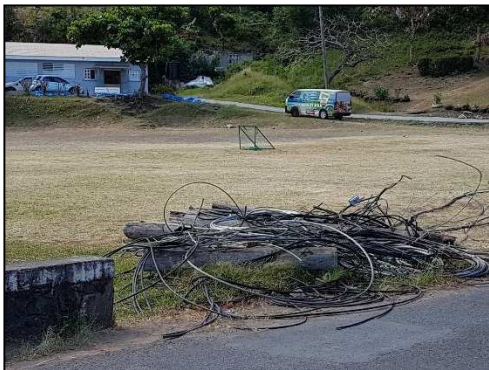
Power lines heaped in a pile. March 2018.
