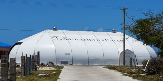
The Samaritan's Purse Operations Hub in Codrington. April, 2018
