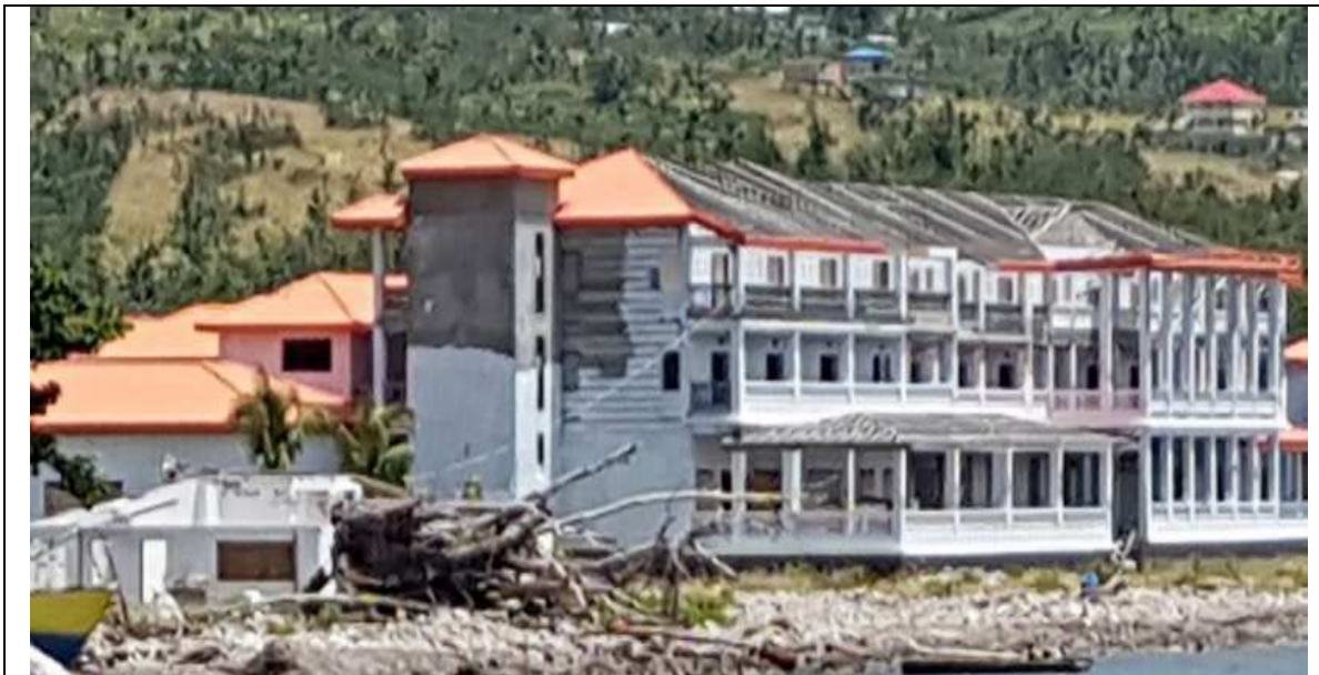
The new Cabrits Hotel Resort and Spa, Portsmouth, March 2018.
