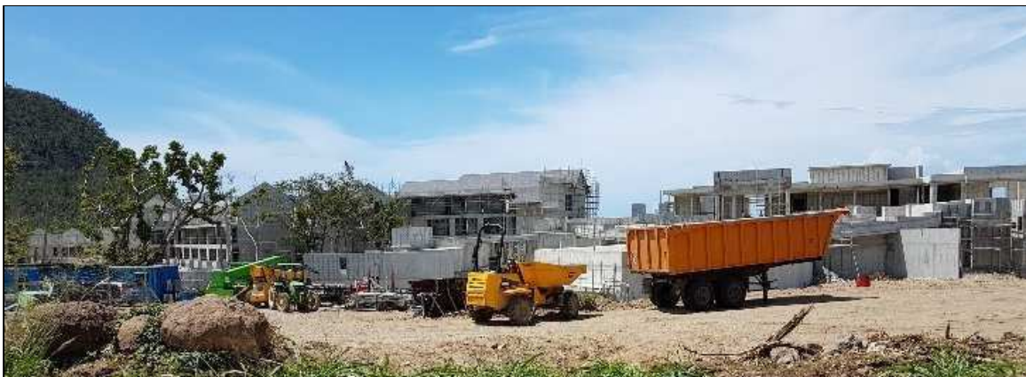
Work continues on the new Anichi Resort and Spa, Portsmouth. March 2018.
