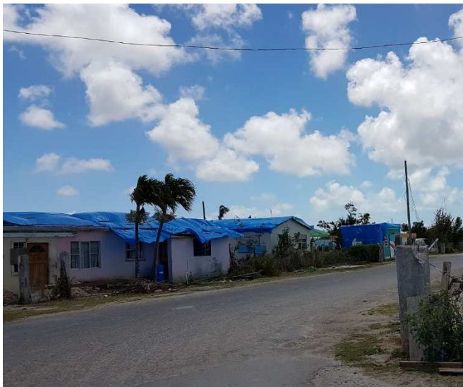
Blue tarps provide roofing, Codrington, Barbuda. April 2018.
