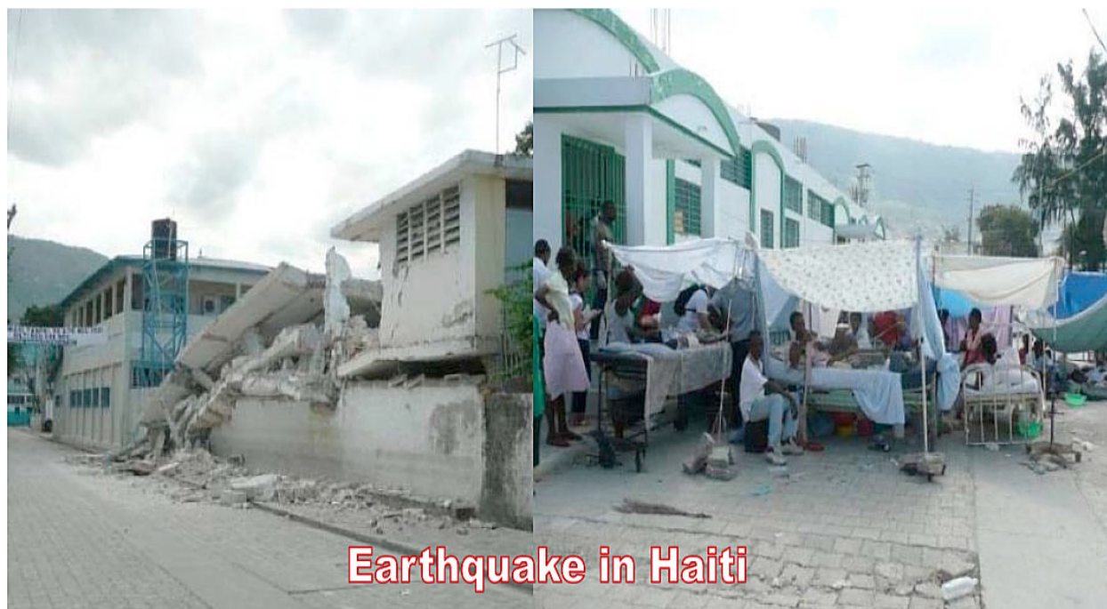
FIGURE 1: IMPACT OF EARTHQUAKE ON INFRASTRUCTURE IN HAITI
