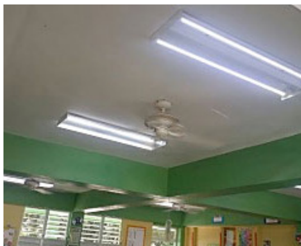
FIGURE 15: INSTALLATION OF ENERGY EFFICIENT LIGHTING
