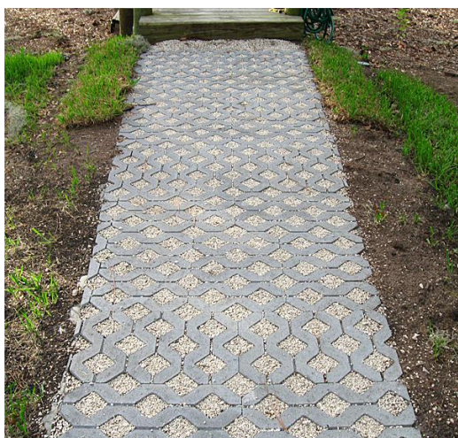
Figure 5: Installed Permeable Pavers
