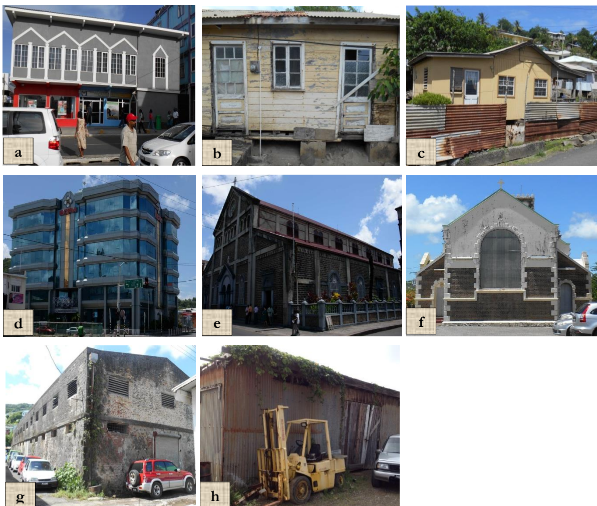
Figure 5-3: Types of wall (a) Concrete block (b) Wood (c) Wood and Concrete block (d) Glass and Concrete block (e) Stone (f) Brick (g) Brick and Stone (h) Galvanized Iron sheet
